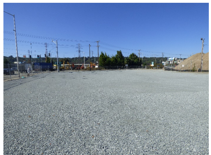
The treatment station site is prepared for construction.
