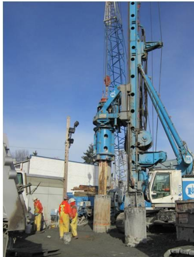
Interlocking secant piles create a ring that will form part of the Influent Pump Station's structural wall.
