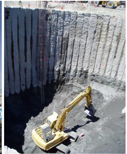
Interlocking secant piles create a ring that will form part of the Influent Pump Station's structural wall.
