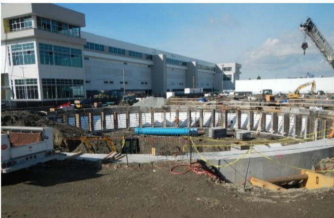
1 Pump station walls on site near the corner of Fourth Avenue South and South Michigan Street (left). The pump station is 45 feet deep and will help bring flows into the station for treatment. Crews are dredging (right) for the regulator station.
