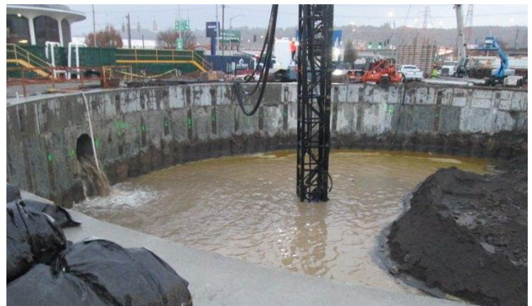
1 Pump station walls on site near the corner of Fourth Avenue South and South Michigan Street (left). The pump station is 45 feet deep and will help bring flows into the station for treatment. Crews are dredging (right) for the regulator station.
