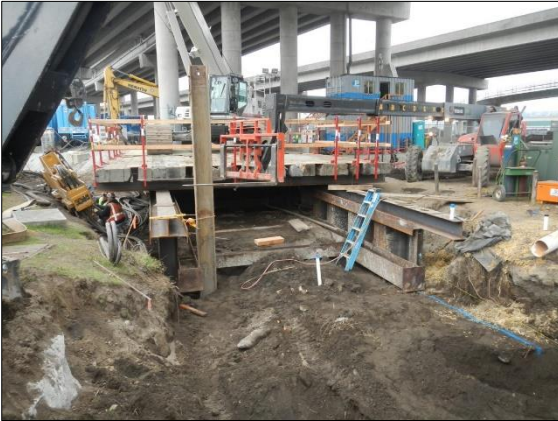
The trestle (shown above) will continue to be installed, eventually moving into the Duwamish River. It will be used to hold the crane and excavator needed for pipe installation.
