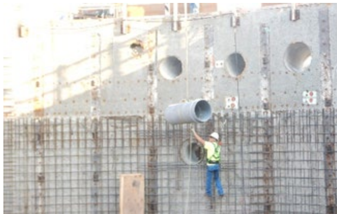
Crew members continue to install steel reinforcements along the walls of the equalization basin.
