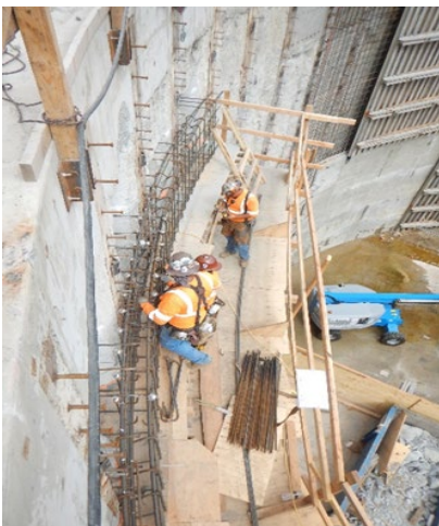
Crew members continue to install steel reinforcements along the walls of the equalization basin.
