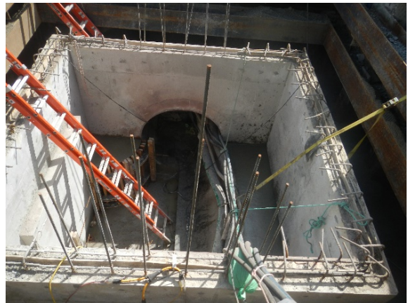
Crews prepare to place concrete infill around the EBI piping.
