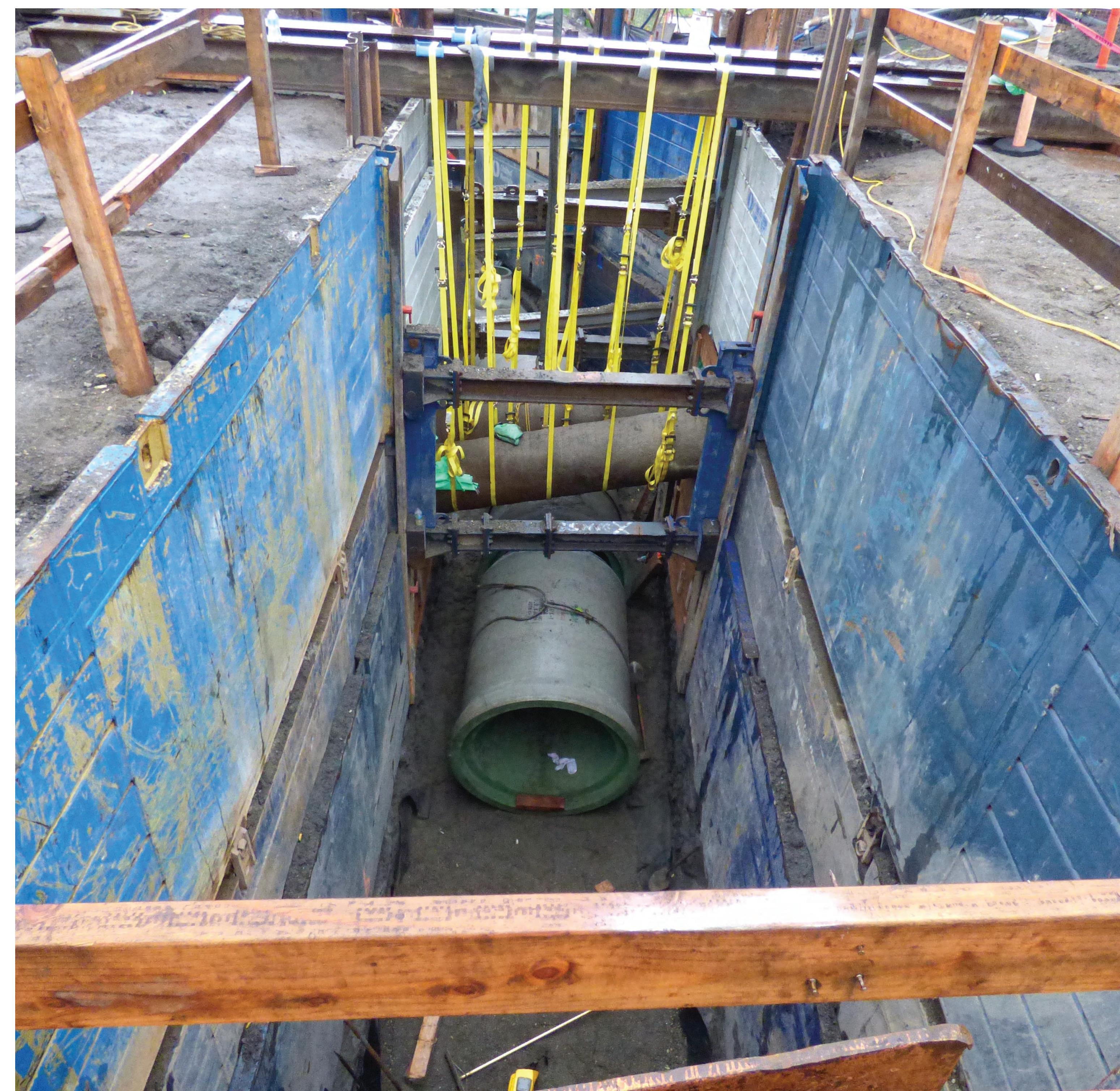
Example of open-cut installation of 60" pipe
