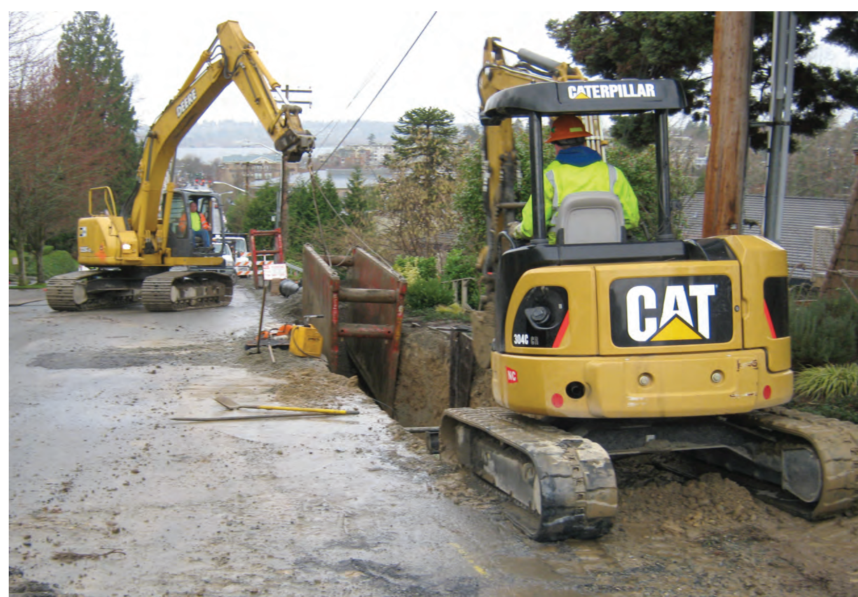
Crews excavate before open-cut installation
