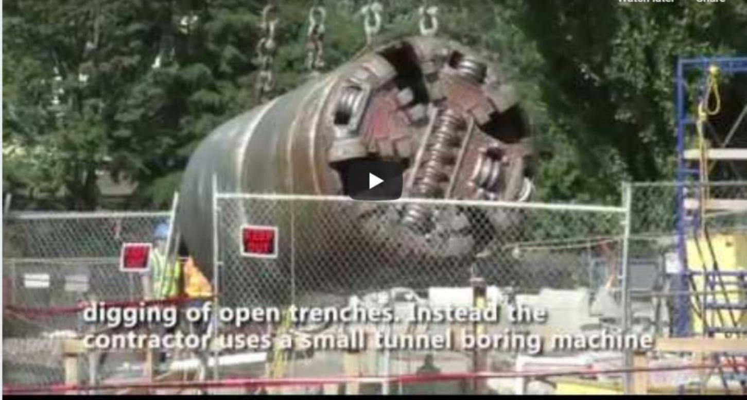
digging of open trenches. Instead the contractor uses a small tunnel boring machine
