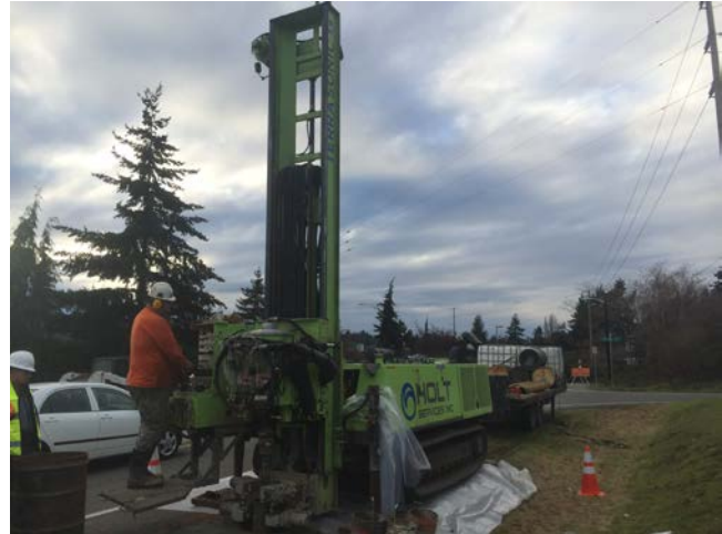
Typical drill rig for work in streets
