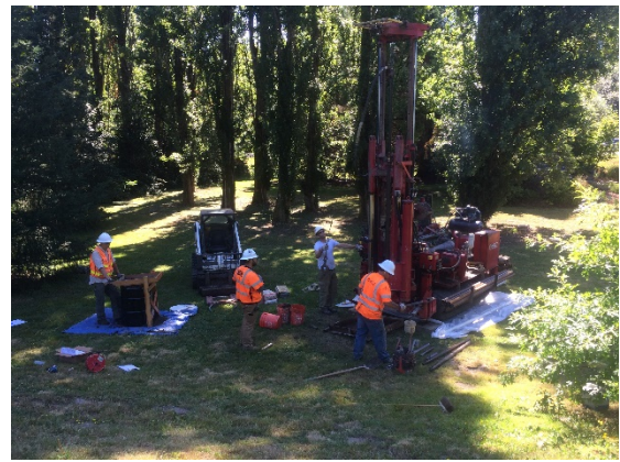
Typical drill rig for soil sampling.
