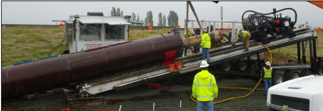
To protect the surface, crews will install steel conductor casings underground prior to drilling the pilot bore.
