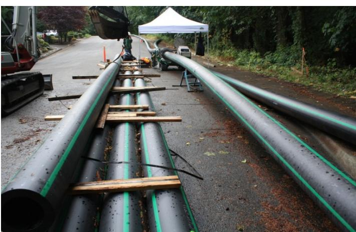
While the drilling crew is preparing the bore hole, a crew uses heat to fuse pipe sections together. The growing pipeline is laid out in long strings. On the day of pullback, the strings are fused together and pulled through the borehole.
