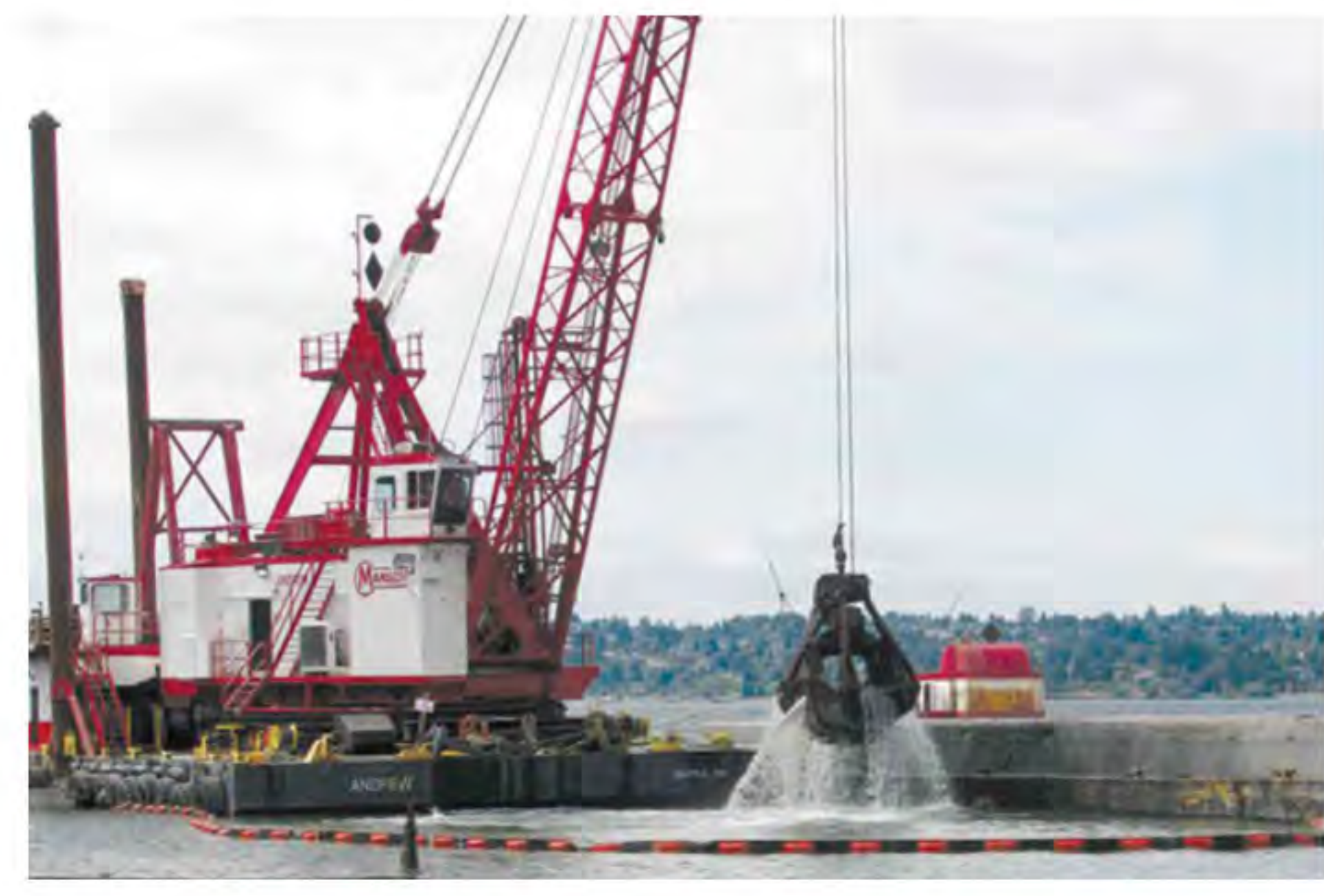
In-water excavation work being performed by a clam shell digger
