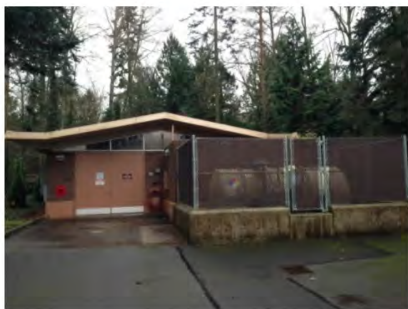
North Mercer Pump Station, located off of S.E. 22nd Street
