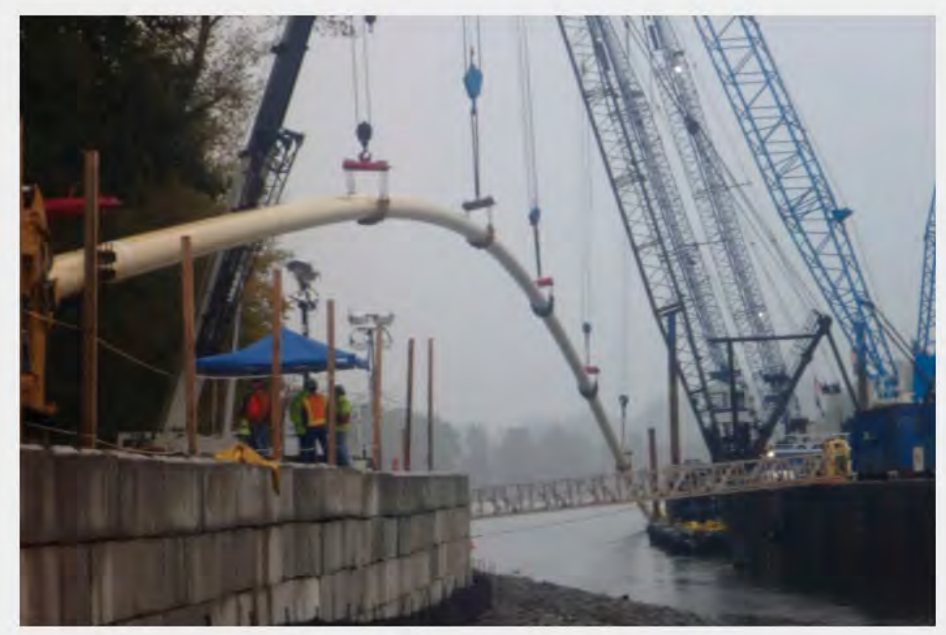
Crews installing a pipe using HDD
