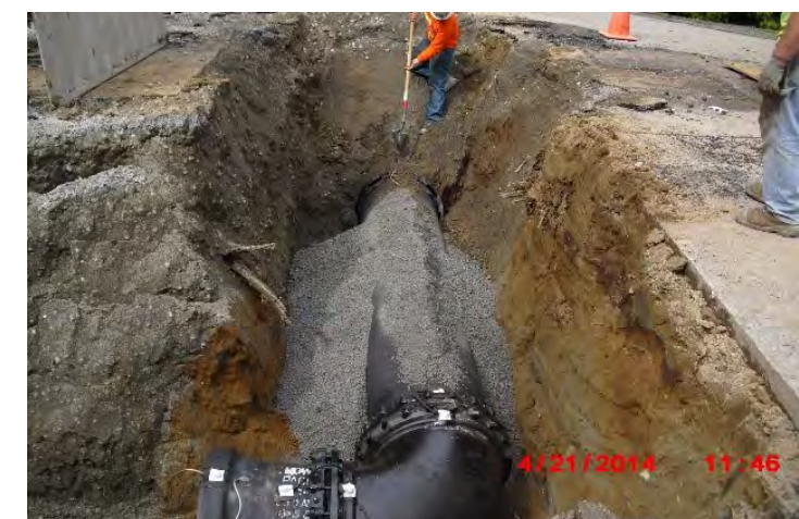
An example of sewer pipe installation in an open trench
