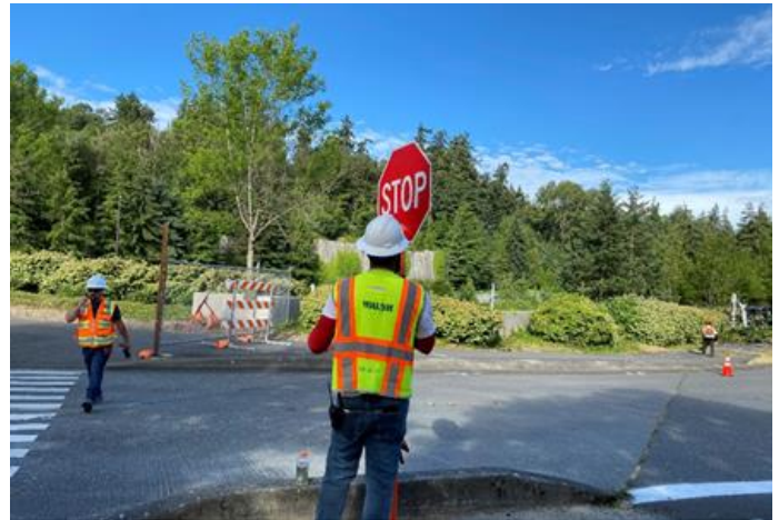
Walsh flaggers direct people to travel through the area safely
