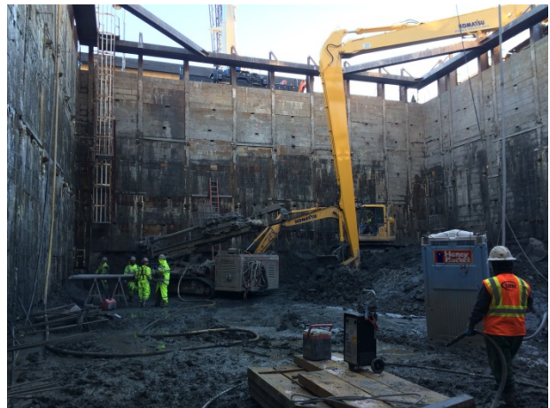
Workers at the bottom of the excavated hole that will hold the storage tank.
