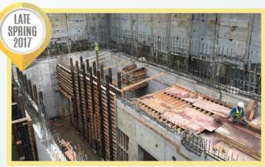
Removable forms were put in place to create the concrete tank walls and internal rooms that will hold the ventilation fans and odor control unit.
