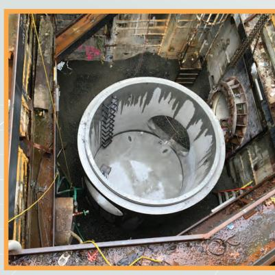
Underneath the access hatch at this location is a large manhole. The manhole connects the new pipes that allow King County to divert wastewater from the pipeline in Rainier Avenue to the pipeline in Bayview St.
