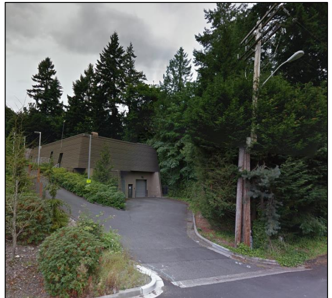
Utility upgrades at the Heathfield Pump Station begin on Wednesday, June 29.
