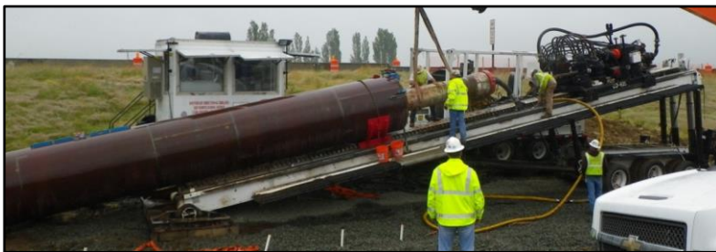
Crews will install steel conductor casings (left) before drilling the pilot bore (right).
