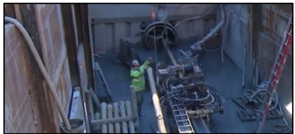
Crews will install steel conductor casings (left) before drilling the pilot bore (right).
