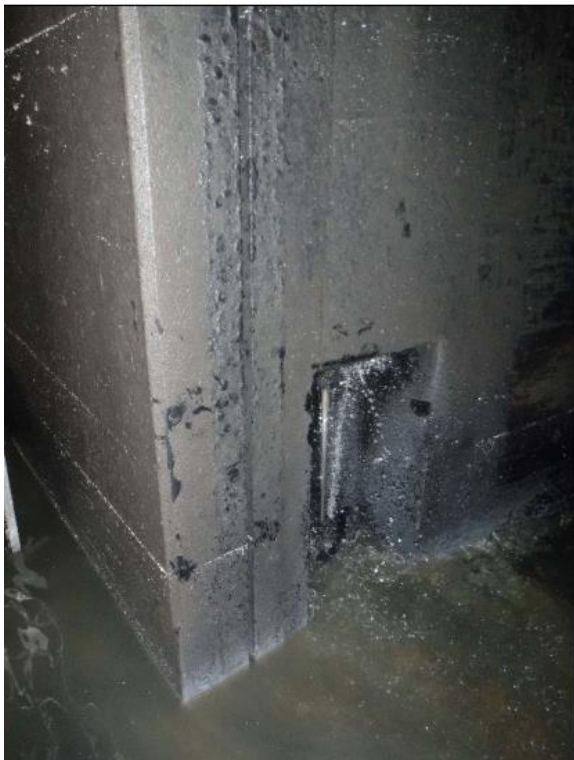
Figure 3-5: 6-inch channel drain system sluice gate at RSP 404
