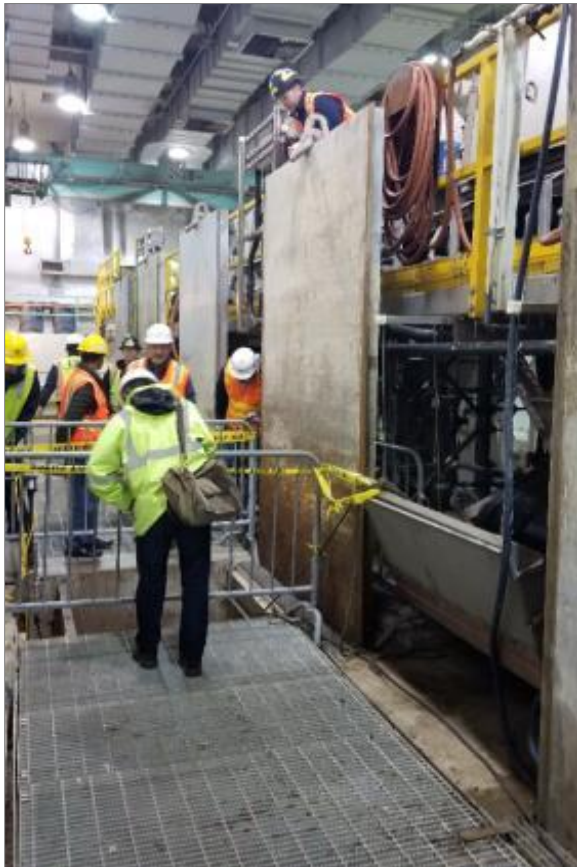
Figure 3-4: Bar screen discharge side isolation slide gate
