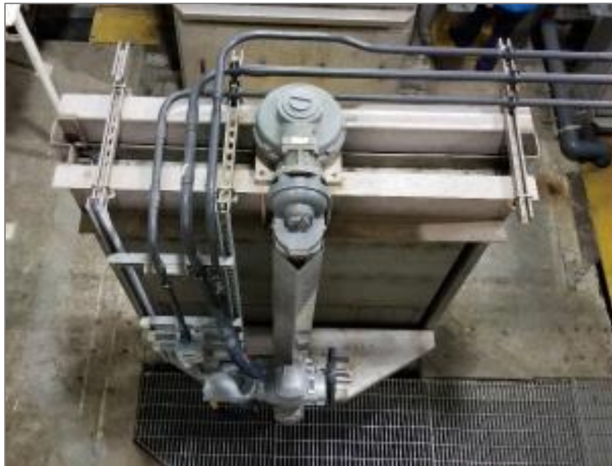
Figure 3-3: Bar screen influent side isolation slide gate
