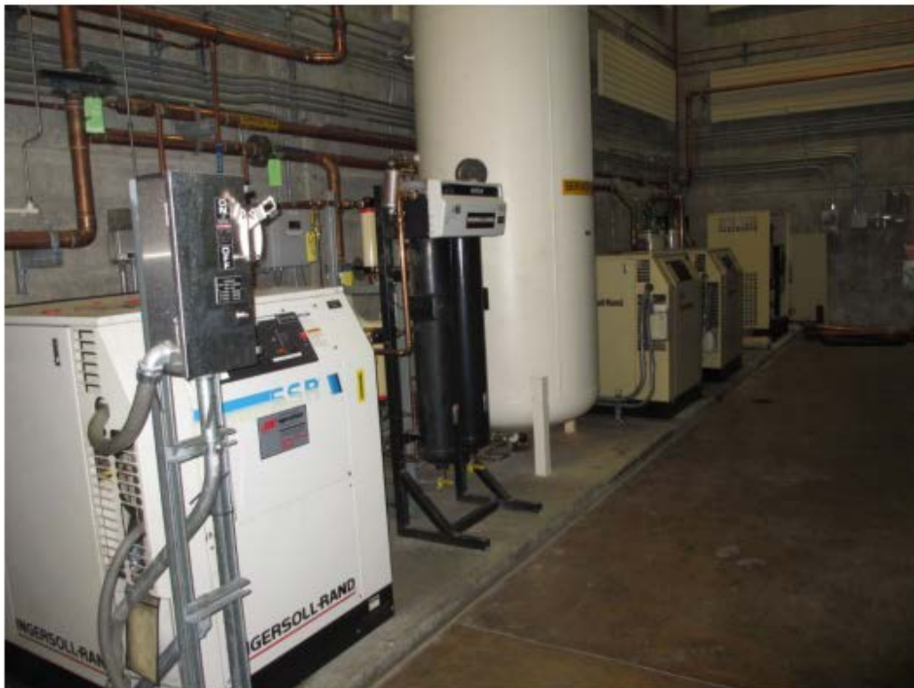
OGADS Air System- Compressor 2 – Dryer #3 - SA Receiver
