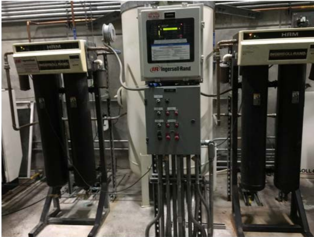
Desiccant Air Dryer Towers Nos. 1 & 2
