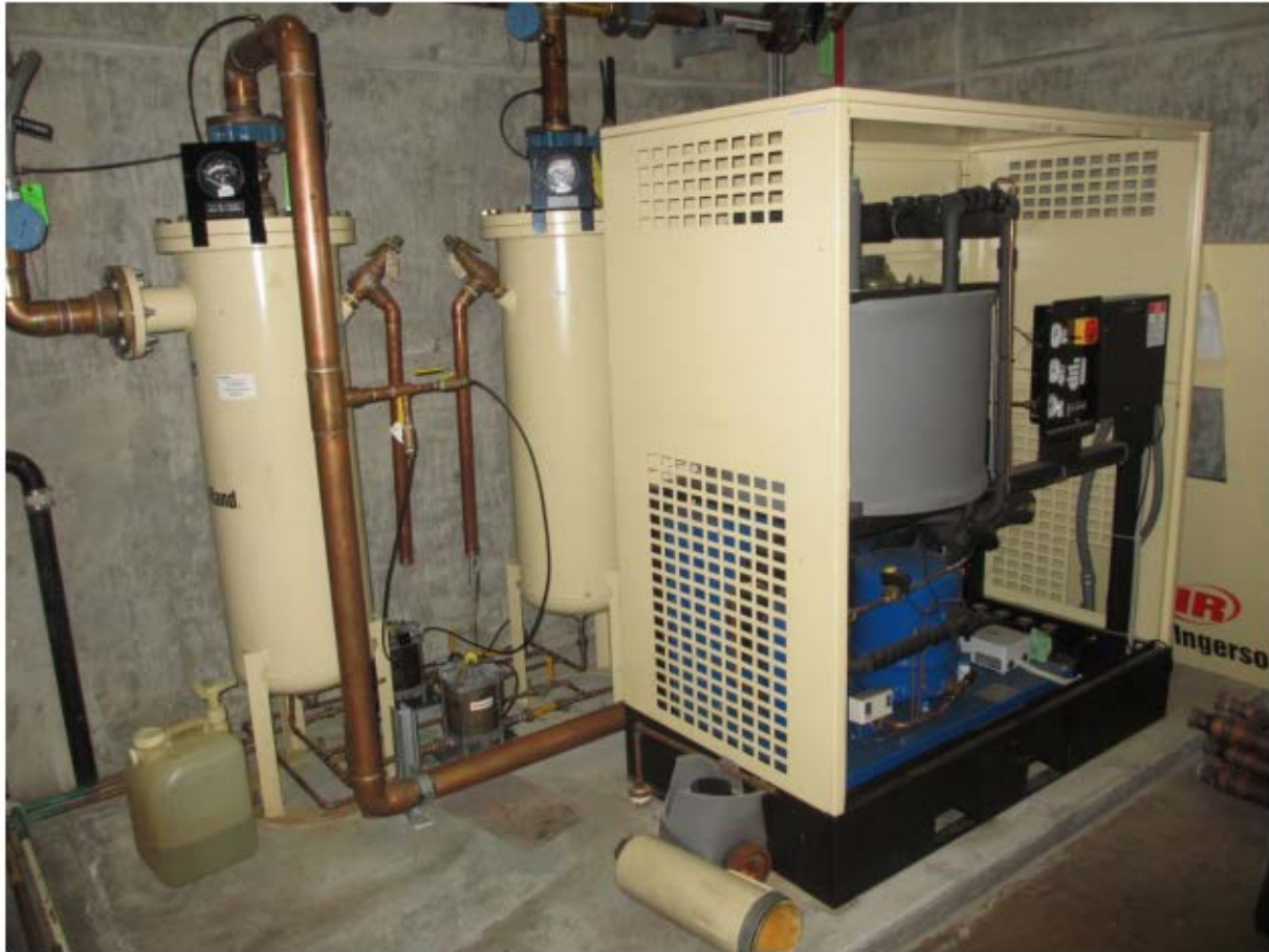
Old Refrigeration Dryer [removed]
