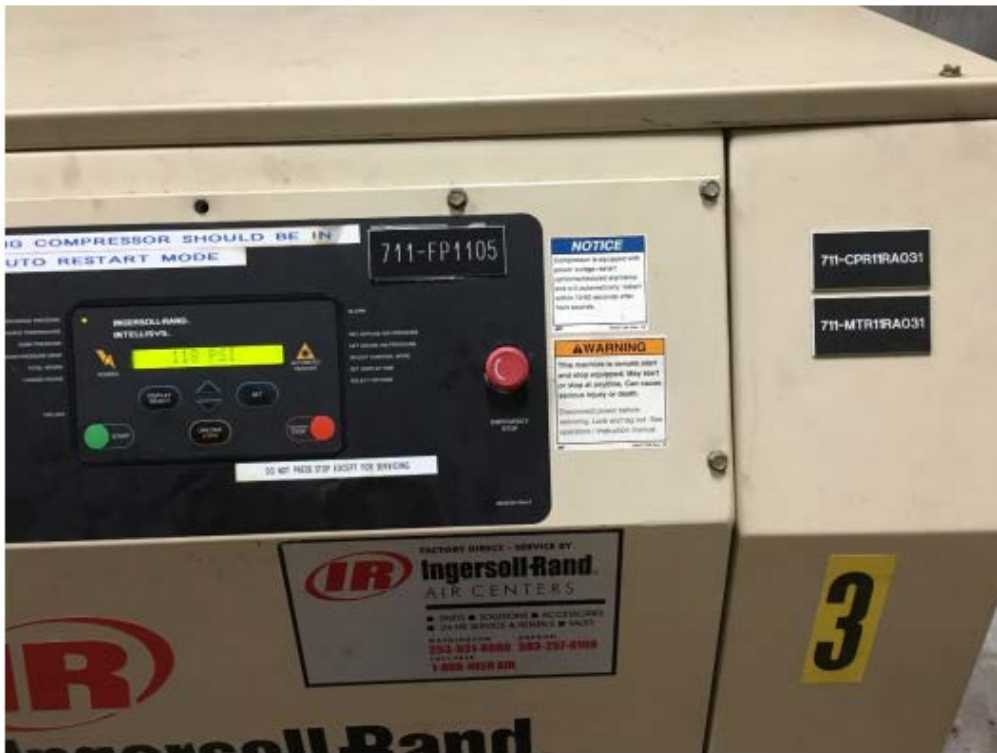
Rotary Screw Compressor 3 Panel Face
