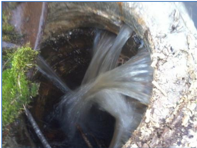
Stormwater inflow into a manhole
