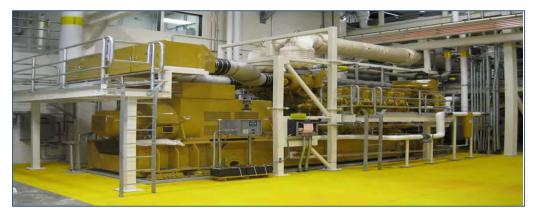
Figure 18. West Point Treatment Plant Cogeneration System
