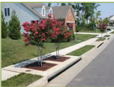
Filterra tree boxes use a small area to capture a high volume of runoff.
