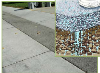
Permeable paving in green alleys allows stormwater to seep into the ground.
