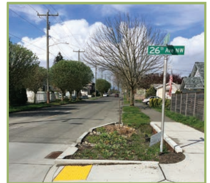
Bioretention can be installed within a curb bulb that also slows traffic.
