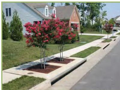
Filterra tree boxes use a small area to capture a high volume of runoff.
