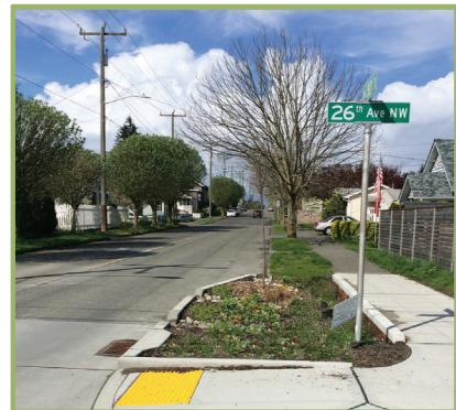
Bioretention can be installed within a curb bulb that also slows traffic.
