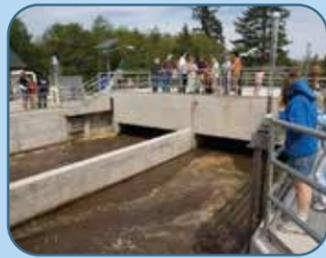
Wastewater **travels** to a tank where microorganisms and bacteria **eat** organic material and contaminants.
