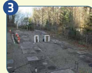
3 Sewage is treated using a series of sand filters and septic tanks. Pollutants settle out in the tanks. Solid material is consumed by good bacteria in a sand filter. UV light is used to disinfect treated water.
