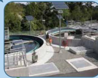
Wastewater goes to big tanks where the solid material **settles** to the bottom of the tank, leaving clear water at the top.
