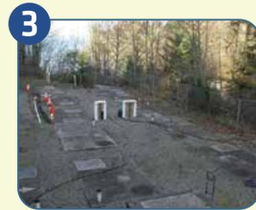
3 Sewage is treated using a series of sand filters and septic tanks. Pollutants settle out in the tanks. Solid material is consumed by good bacteria in a sand filter. UV light is used to disinfect treated water.
