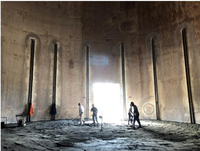
2019: The District installed steel stiffeners inside the 2 MG tank to provide stability during seismic events. Note the size of the workers for scale.
