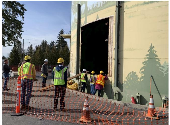
2019: American Water Works Association Young Professionals take a tour of the 2 MG tank seismic retrofits. The contractors conducted all work through a large access point cut into the wall of the steel tank.
