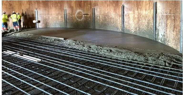
*2019: Seismic retrofits at the District’s 2 million gallon tank included the pouring of a concrete pad and installing steel stiffeners on the inside walls.*
