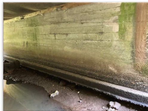
Scour under abutment footing at SE 408th Street Bridge No. 3056A
