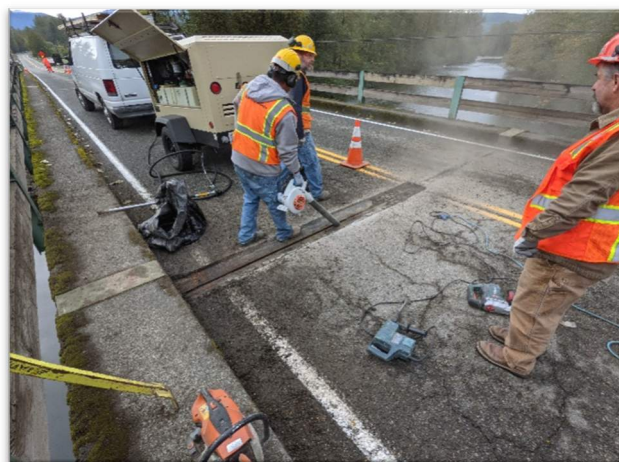
Expansion Joint Repairs at North Fork Bridge No. 122i
