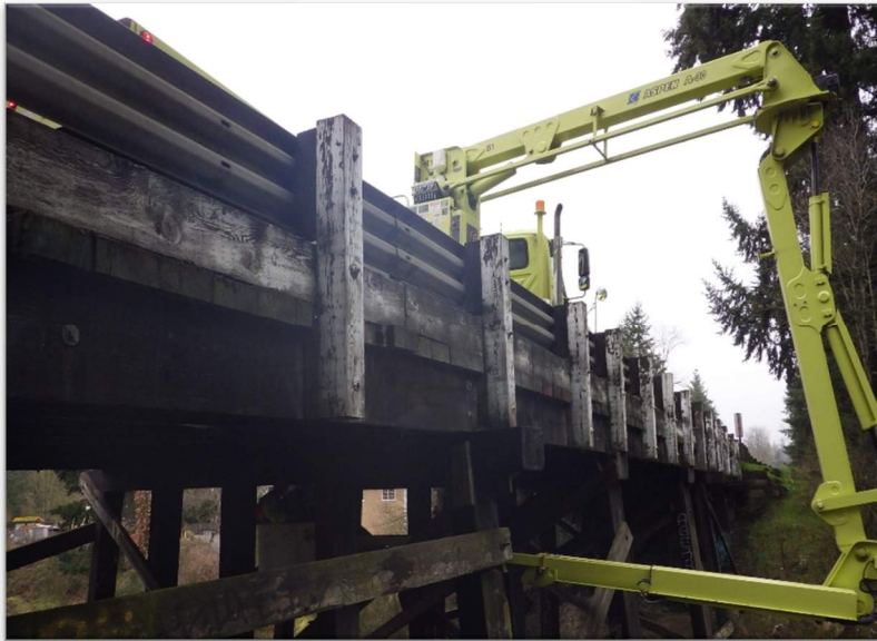
Berrydale Overcrossing No.3086OX with an Under Bridge Inspection Truck (UBIT)
