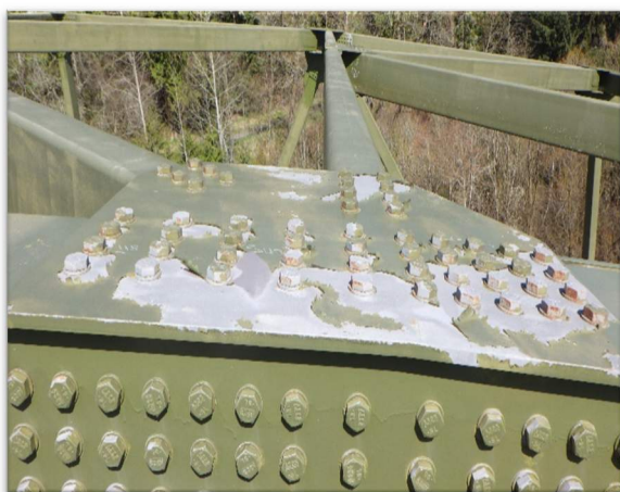
Peeling paint on upper gusset plate at Tolt Bridge No. 1834A
