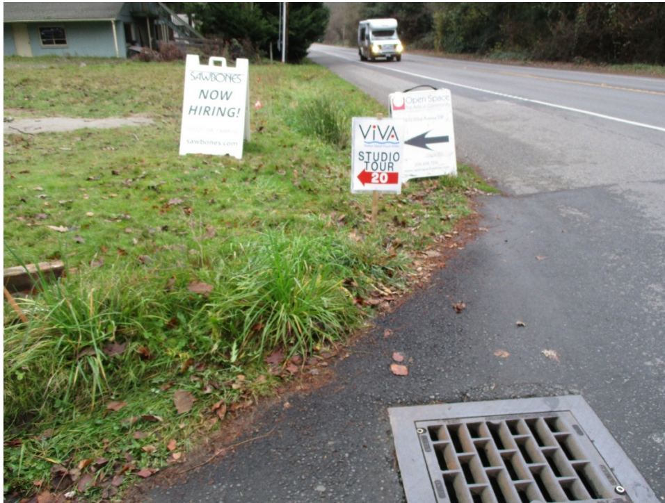
Figure III-4 Vashon Hwy looking north, CB picks up north half of runoff of 188 th (proposed site towards west).
