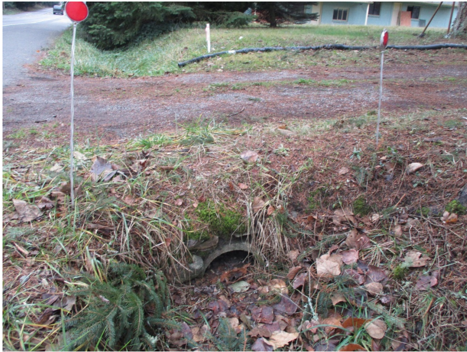
Figure III-6 Culvert at neighboring driveway (looking south towards site), neighbors HDPE pipe connecting to ditch.
