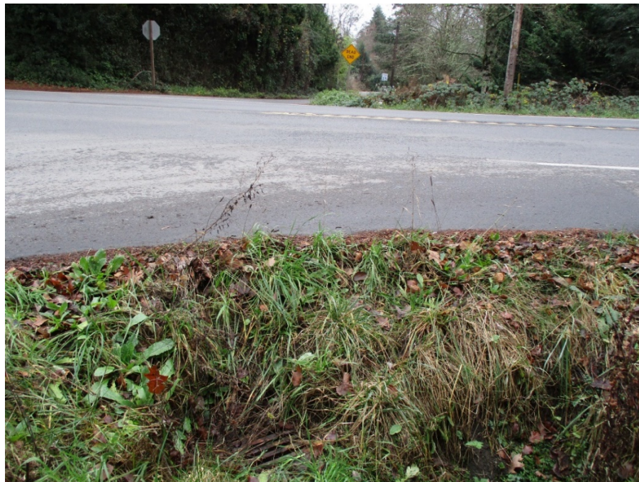
Figure III-3 Vashon Hwy looking east at intersection of Vashon Hwy and 188 th . CB on west site of street picks up half of runoff off 188 th .
