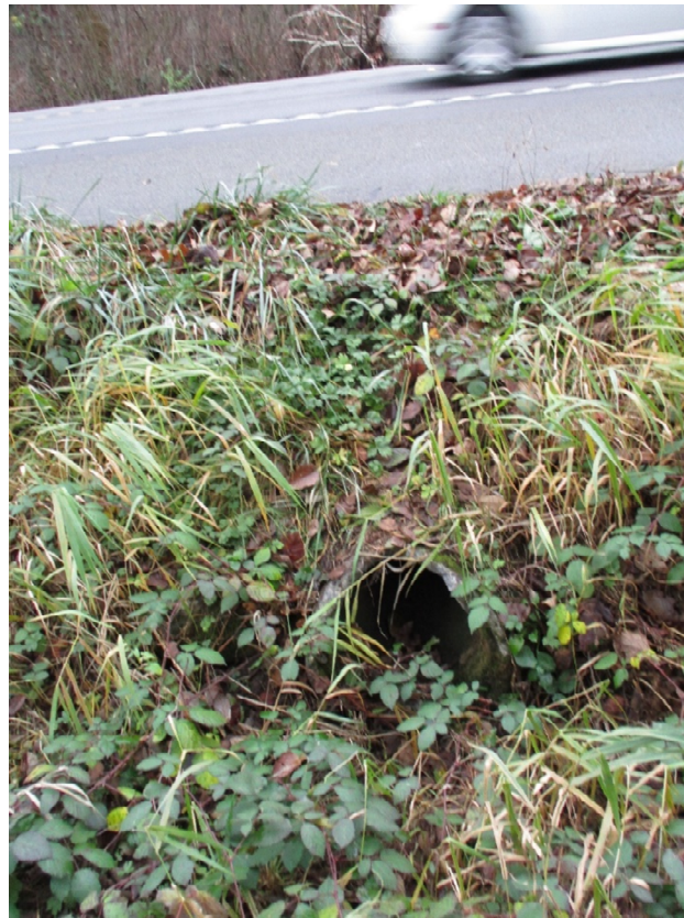
Figure III-9 24" Culvert within ditch line crossing Vashon Hwy, looking east.
