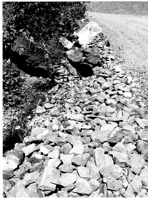
Culvert Conveyance: The mining operation conveying storm waters towards the settling/detention ponds.
