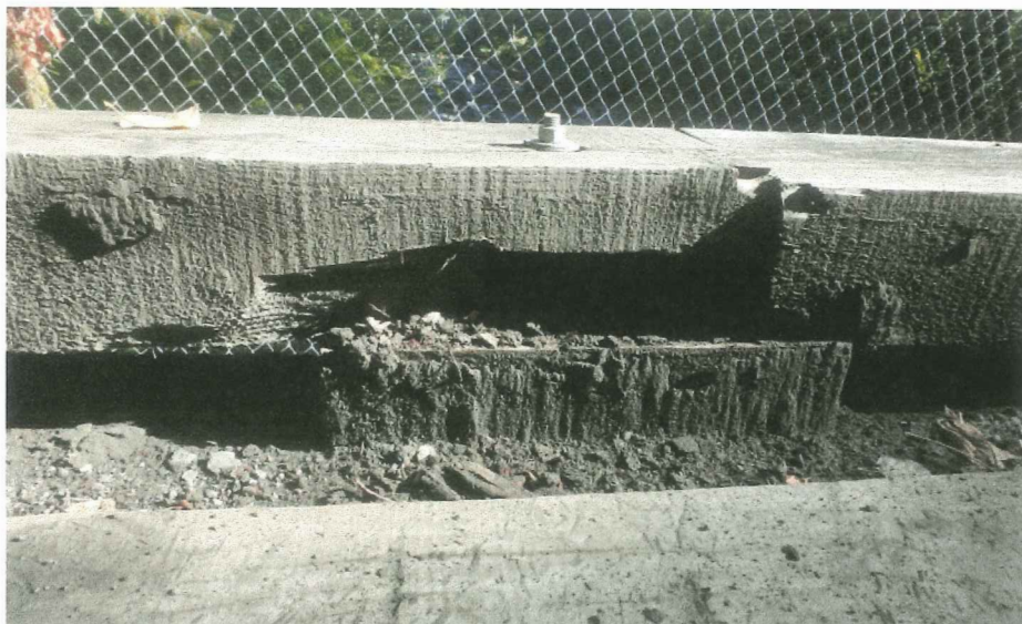
Photo 4 – Dry rot damage in timber curb member
