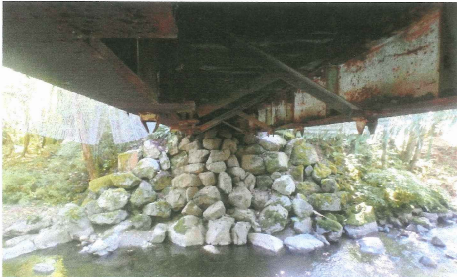
Photo 6 – Diaphragms made from steel angles. Note the cover plate welded to the bottom flange of the girders. Also note the good condition and distribution of the armor rock at the east abutment.
