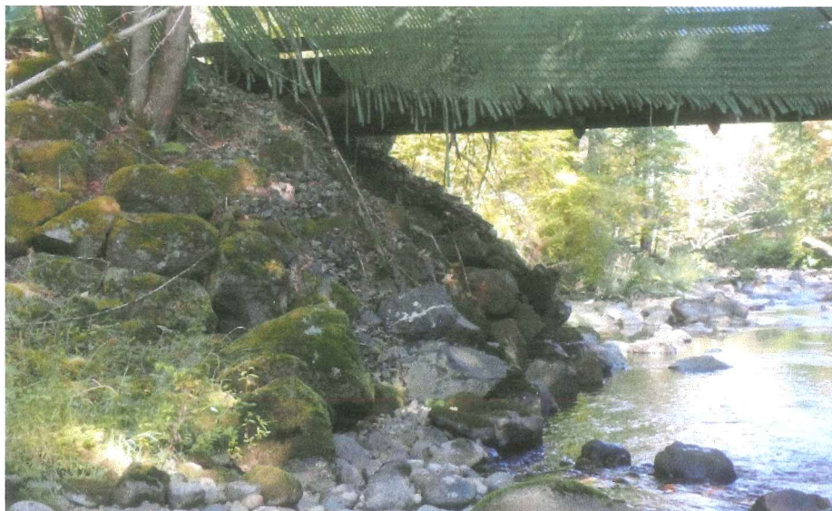
Photo 6 –View of the armor rock at the upstream side of the west abutment. The riprap is in good condition.
