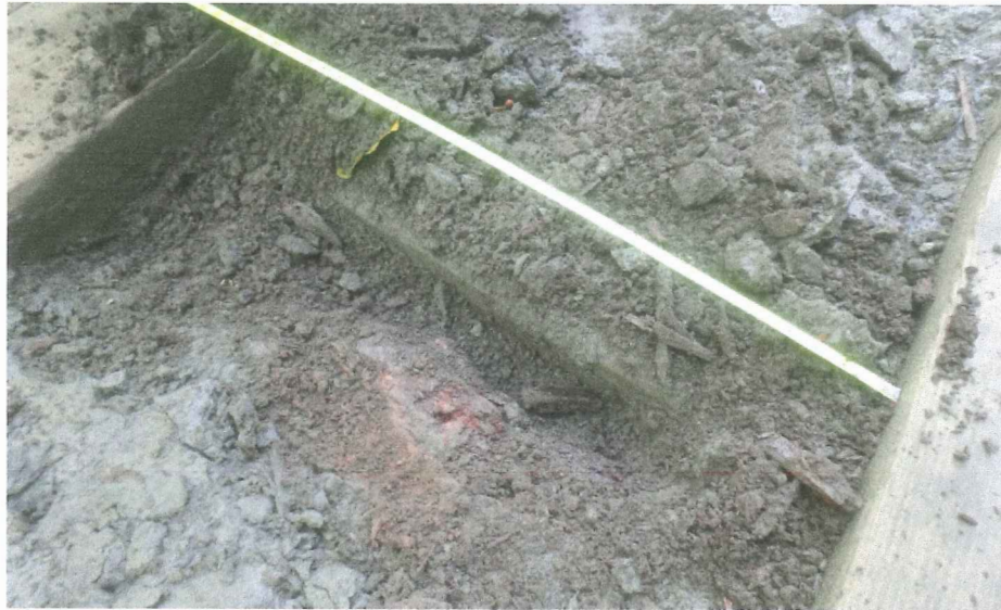
Photo 3 – Dry rot damage in transverse timber deck member
