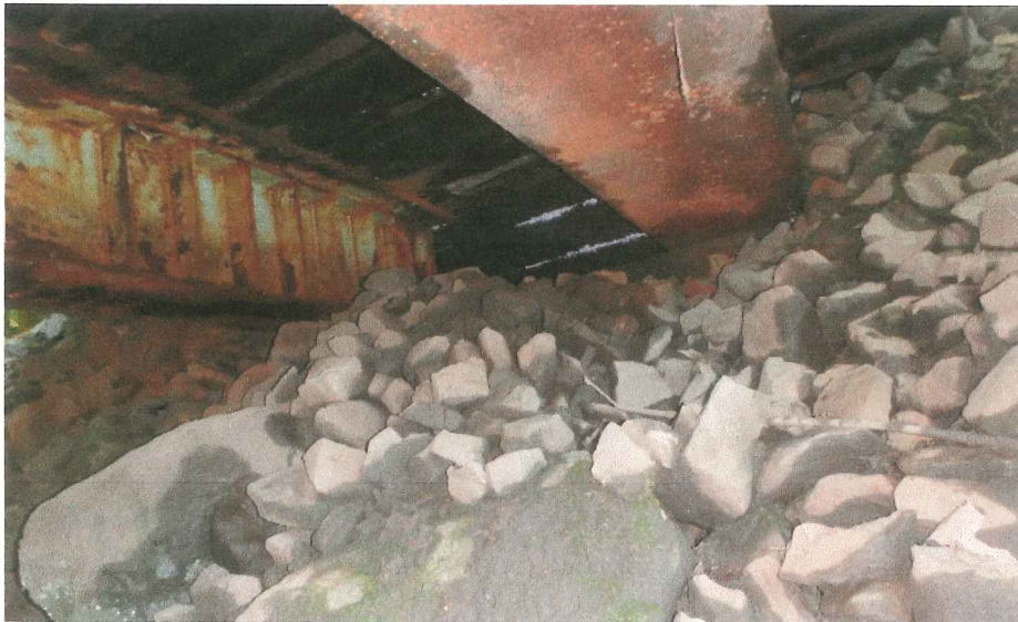
Photo 5 – View of the west abutment. Note the quarry spalls which have been added since the previous inspection.
