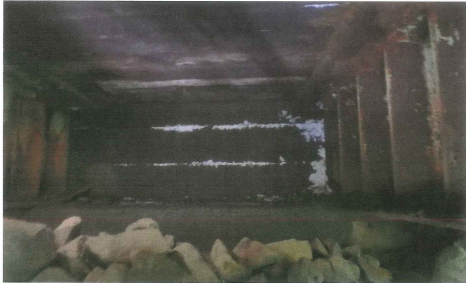
Photo 5 – West end of the bridge. Note the web stiffeners welded to the girder, the lack of bearings, the concrete spread footing, and the timber back wall.
