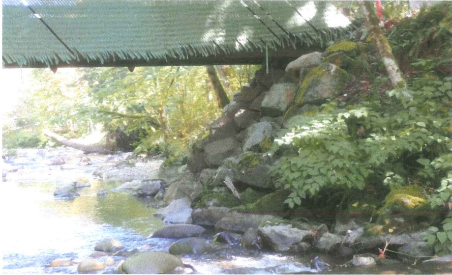
Photo 4 – Armor rock protection at the upstream side of the east abutment is in good condition.
