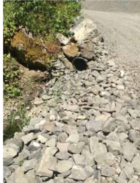
Culvert Conveyance: The mining operation conveying storm waters towards the settling/detention ponds.
