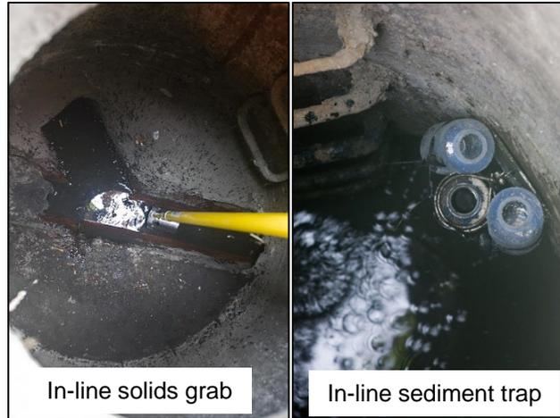
**Figure E-1. Example of In-line Solids Grab Samples and In-line Sediment Traps**
