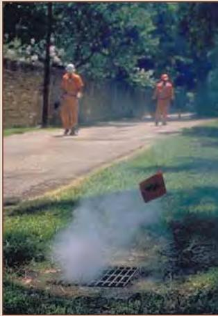
**Smoke Testing** involves pumping smoke through sewers from manholes in streets and observing where smoke exits. The exiting smoke can indicate a broken pipe or where roof or foundation drains might be illegally connected to the sewer system.
