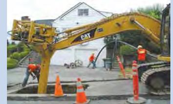
Pipe bursting is a technique that pulls a hardened steel breaker head through the old pipe, breaking it up, and replacing it with a new pipe all in one process.
