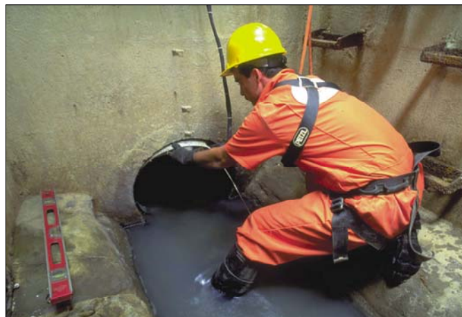
Figure C2 Installation of Open Channel Area-Velocity Metering Equipment
