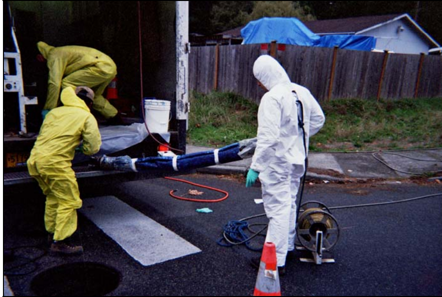
A 4-foot section of blue liner wrapped around a packer in preparation for a CIPP spot repair. Blue resin is fast curing epoxy.
