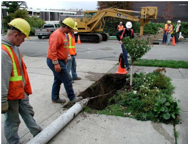
Pipe bursting of a lateral. Pull was approximately 40 feet long.
