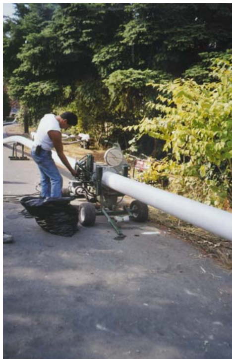
Gray HDPE sections being welded into long lengths.
