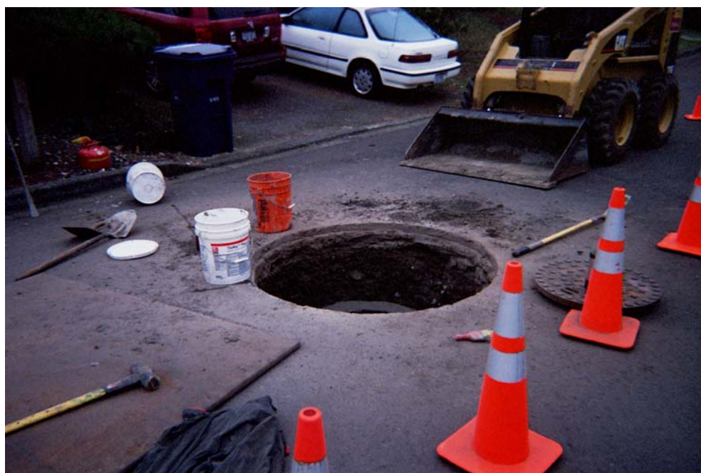
Manhole with lid, frame, and leveling rings removed; ready for WHIRLyGIG installation.
