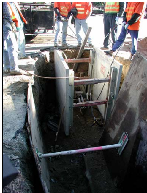
Figure 7-19. Pipe Bursting 5
