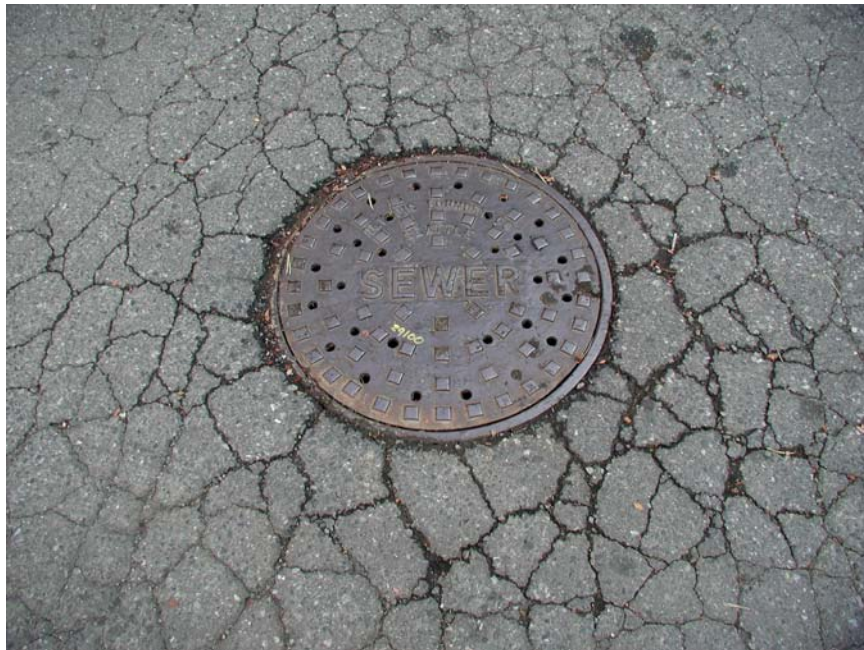
Manhole with indications of settlement in the pavement that likely subject the cover to inundation during rainfall. The large number of pick holes in the lid also allows free flow of surface water into the manhole.
