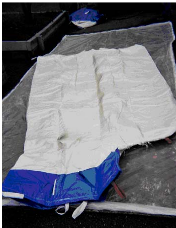
Fiberglass manhole liner prior to wet-out.
