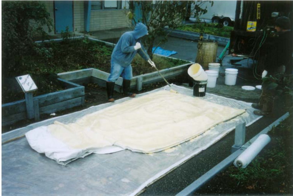
Fiberglass manhole liner being wet-out in the field.
