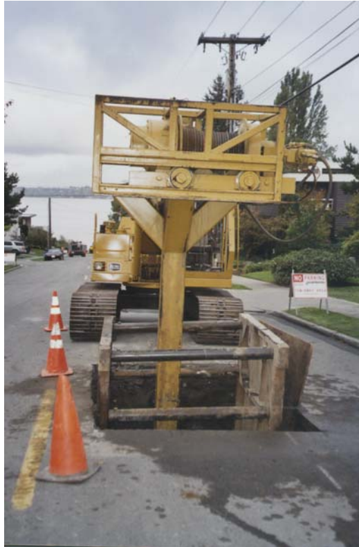
Trackhoe positioned at pulling pit during pipe bursting.
