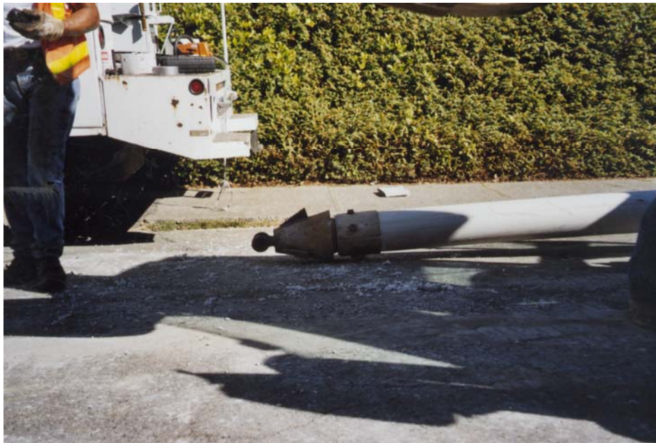
Pipe bursting head attached to an 8-inch-diameter HDPE pipe. Note extra fins.
