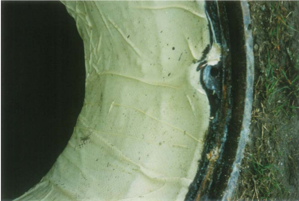
Fiberglass manhole liner trimmed at the manhole ring.
