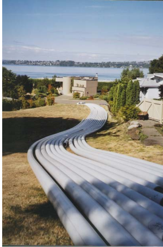
Sections of welded HDPE ready to be dragged into position.
