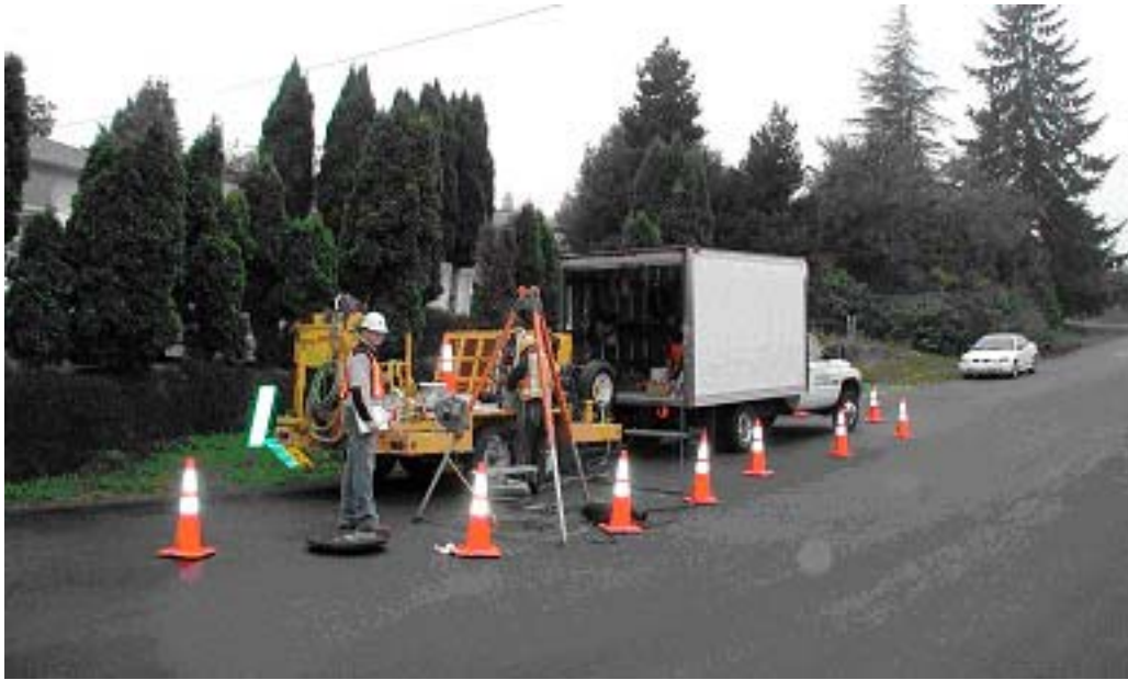
Chemical grouting operation for manholes.
