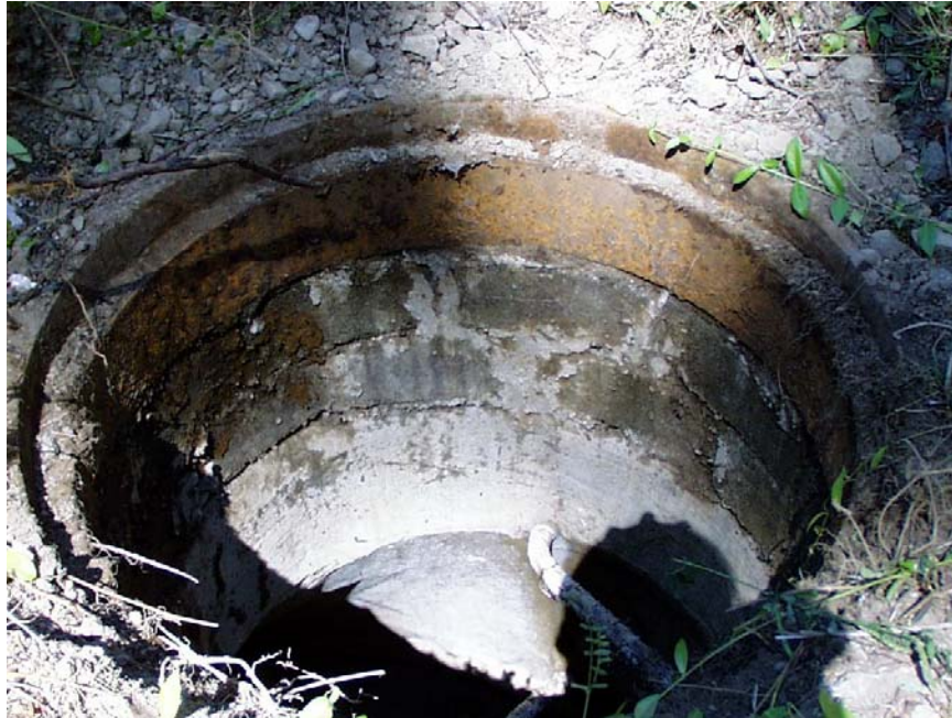
Manhole chimney in need of repair.
