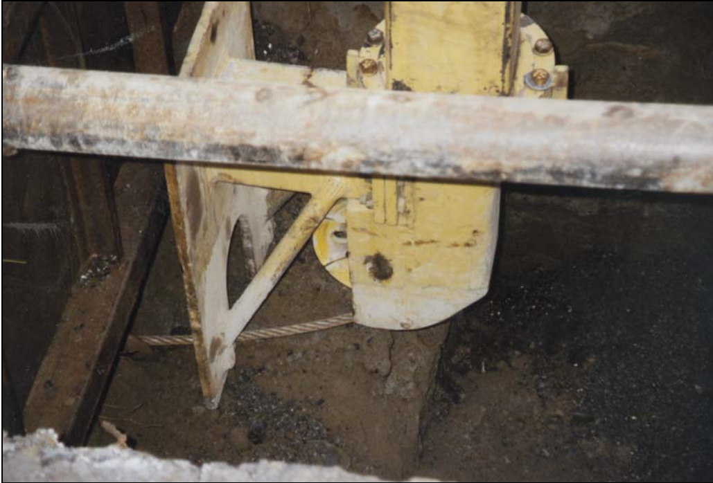
Pipe bursting pressure plate and cable ready to begin pull.
