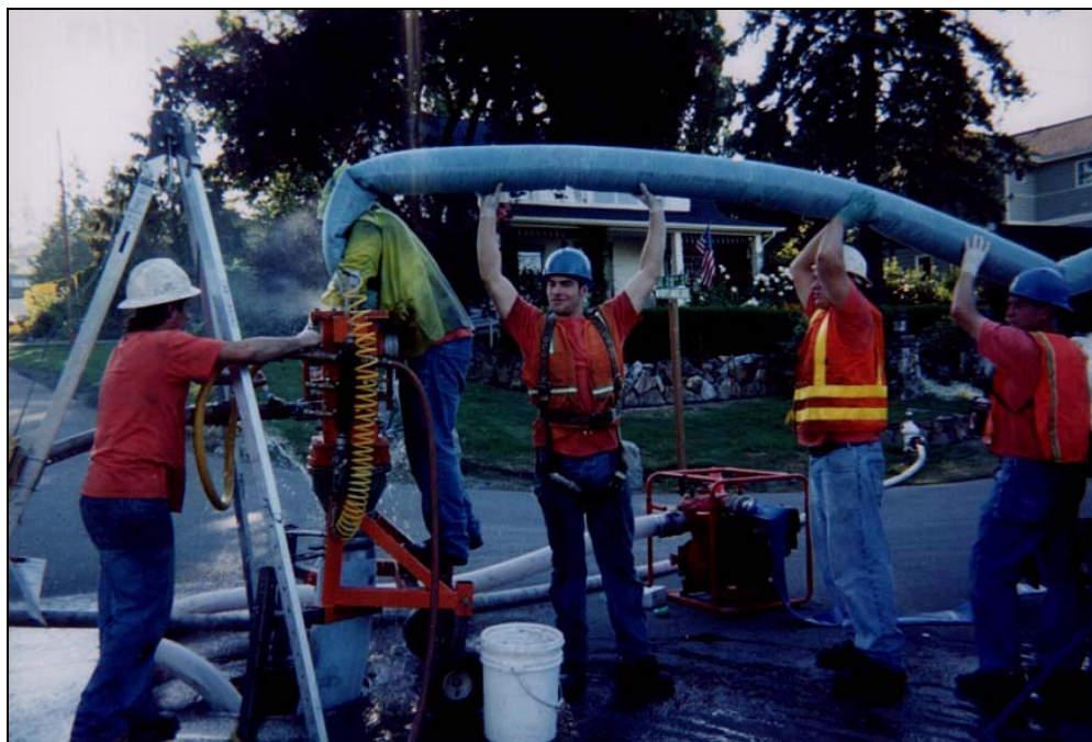
Crew installing CIPP using the air inversion method.
