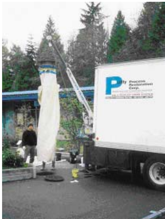
Fiberglass manhole liner being lowered into manhole.
