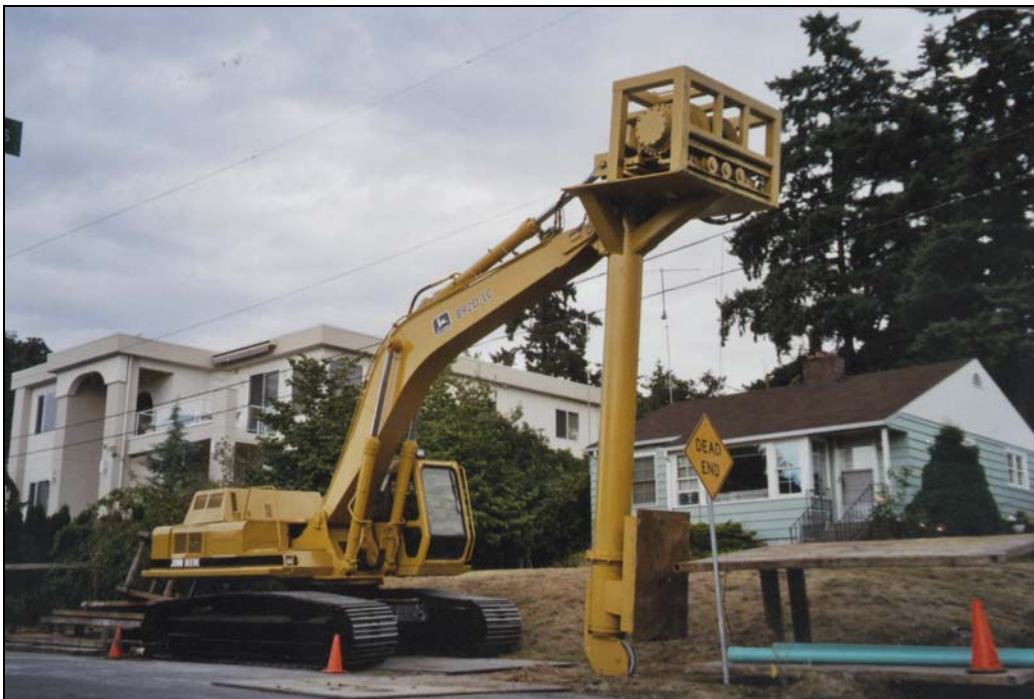
Trackhoe configured for pipe bursting. Note hydraulic motor, boom, and pressure plate.
