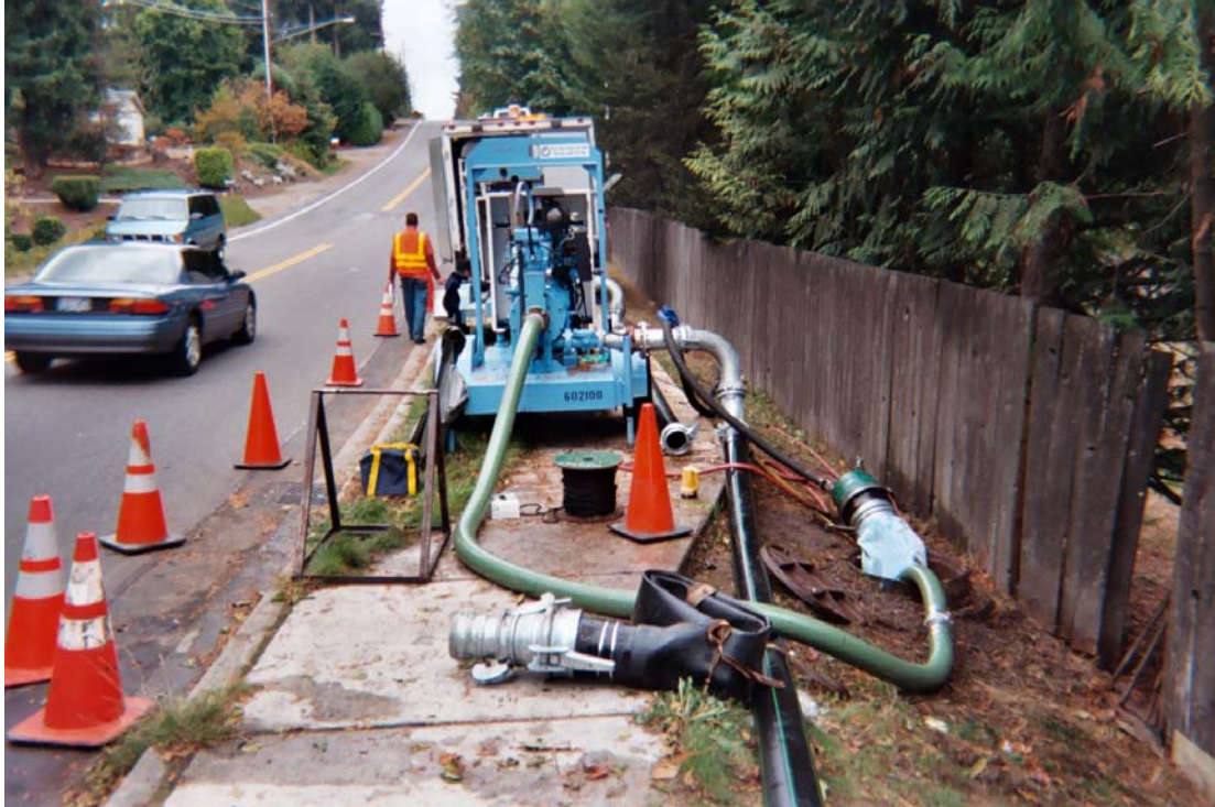
Figure 7-55. Bypass Pumping System
