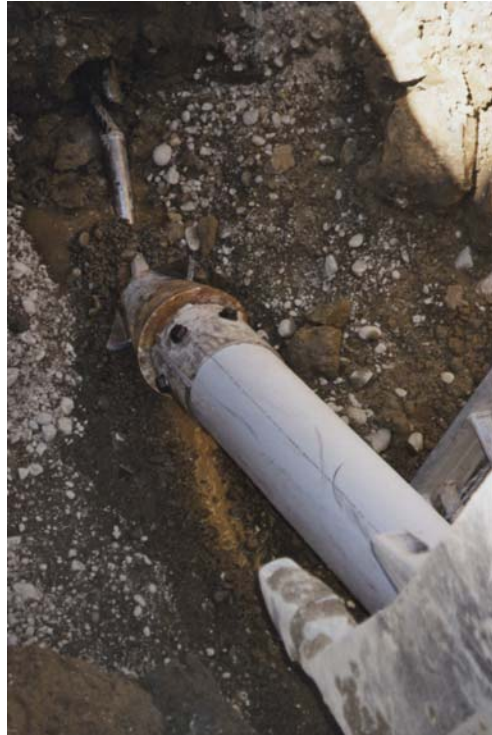
Figure 7-19. Pipe Bursting 5
