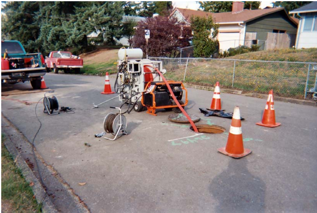
T-Liner® installation equipment located at downstream manhole. Similar equipment is located at the upstream manhole as the liner is placed inside the sewer main.
