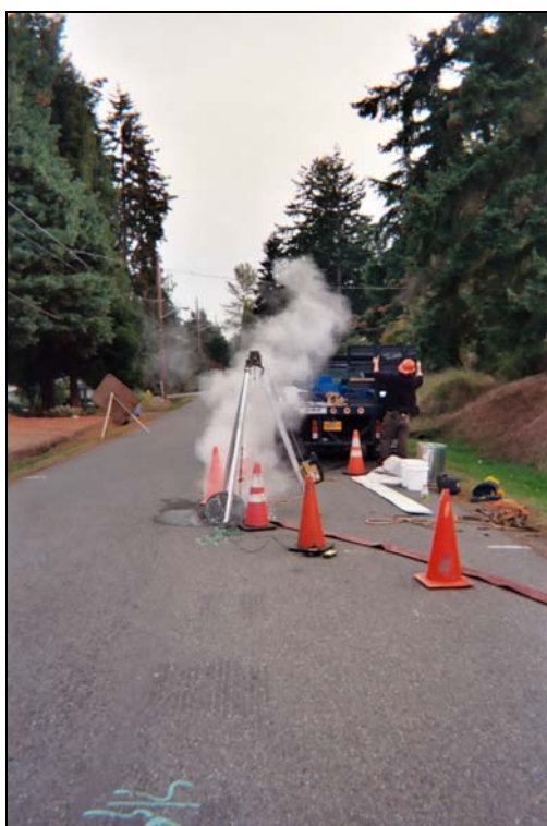
Steam exiting tail end of CIPP during the curing process.
