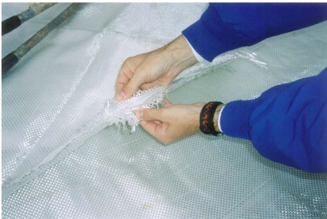
Layering of fiberglass manhole liner prior to wet-out.
