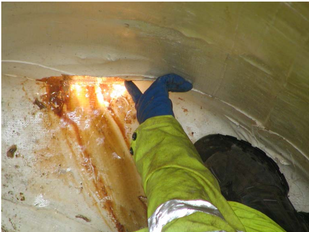
Leak in a cured fiberglass manhole liner.
