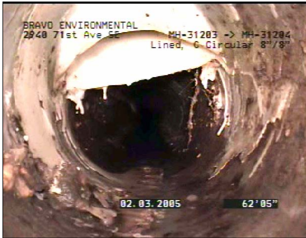
Figure 1 – Homeowner installation of CIP liner in lateral
