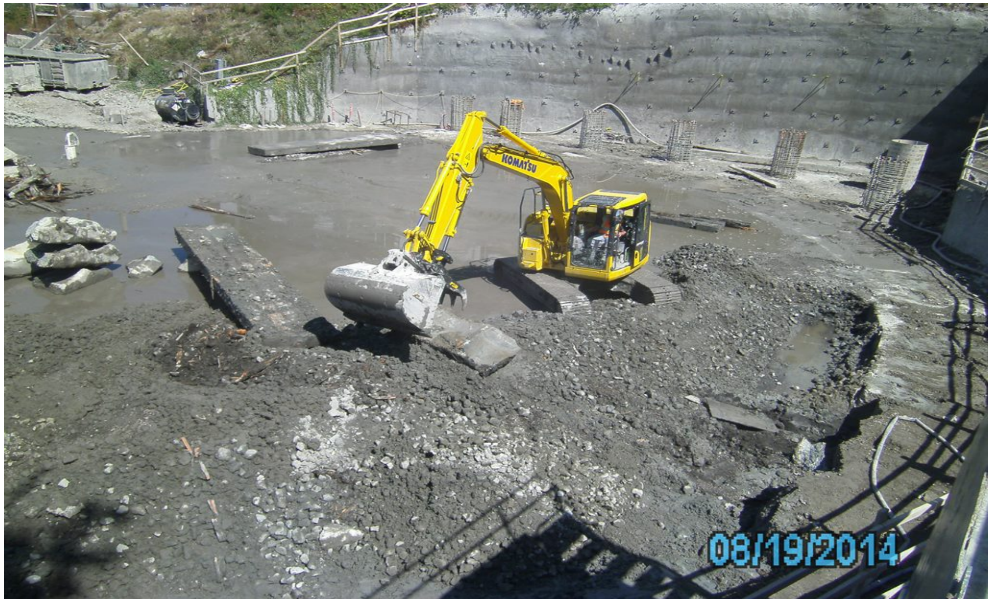
Preparing for dewatering well installation
