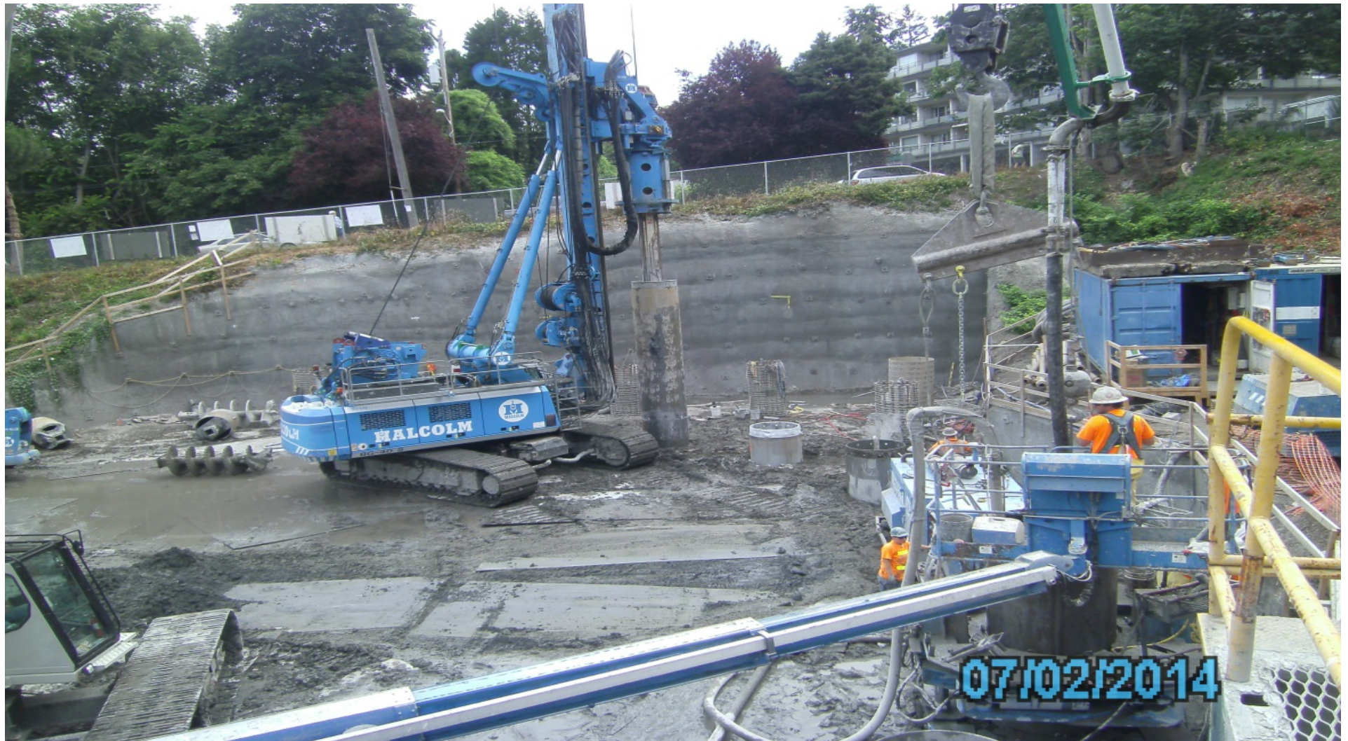
Placing concrete for a secant pile and drilling a second secant pile. 50.1 nail shoring is visible in the background
