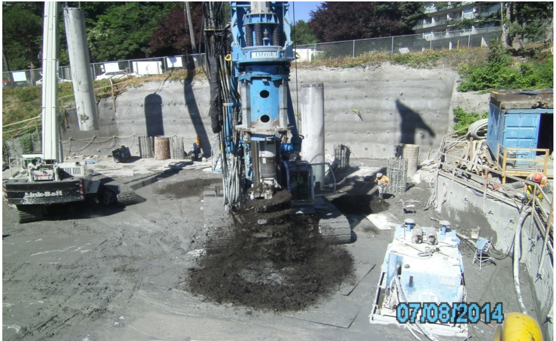
Drilling a starter casing for a secant pile
