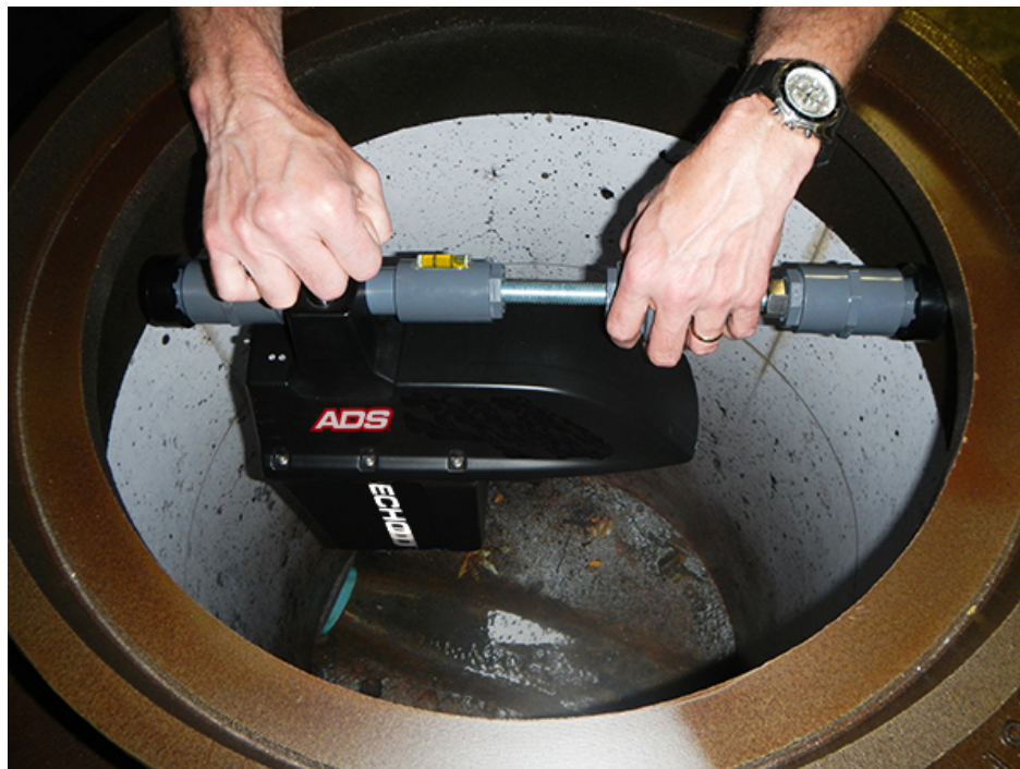
Flow Level Measurement Monitor Example Installation
