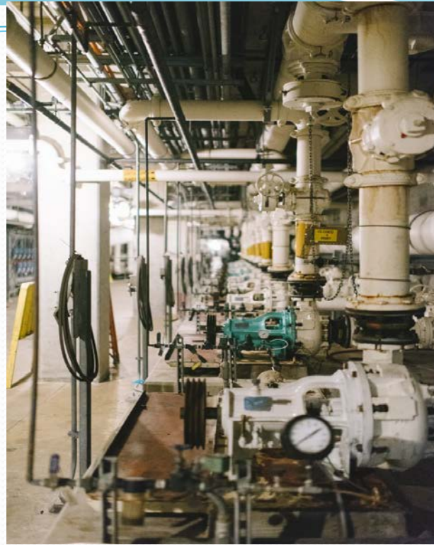
Gravity Belt Thickener Feed Pumps - Ready for replacement motors
