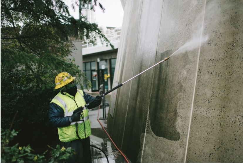
Pressure washing a digester
