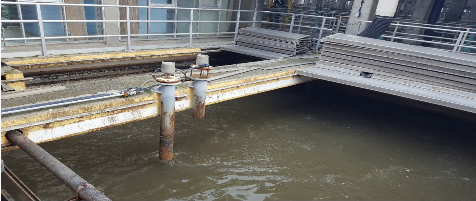
Primary Sedimentation Tanks High and High-High Float Switches
