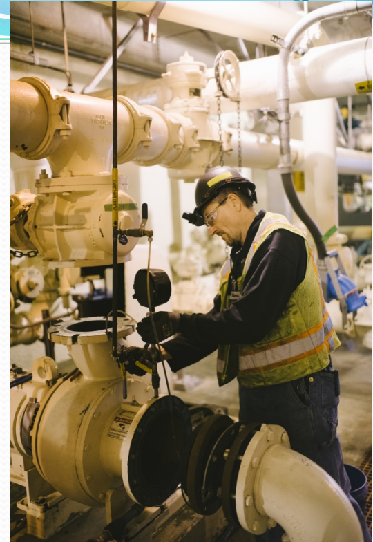
Pumps for Biosolids being repaired
