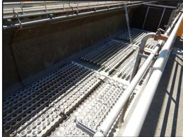
**Figure 2-3. South Plant Aeration Diffuser Membrane Installation**
