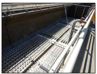
Figure 2-3. South Plant Aeration Diffuser Membrane Installation
