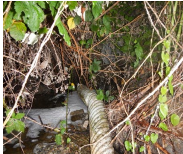
SR4—LOOKING AT SCOUR POOL BY ROADWAY PIPE OUTLET
