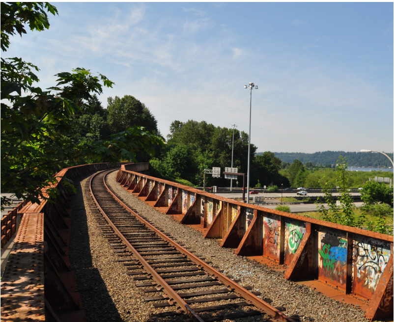
The sidewalls on the ERC bridge crossing I-90 are structural, and cannot be modified. The trail may be developed at the current level of the tracks, but at substandard width, or built at the top of the sidewalls at the full recommended width. Building the trail level with the top of the sidewalls would simplify the future connection to the I-90 Trail.
