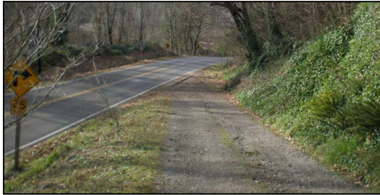
Figure 1.8: Existing Southern Driveway (also referenced in Alternative 2)
