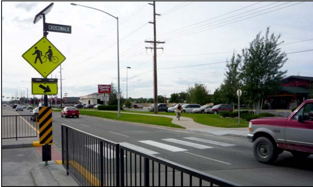
Figure 1.26: Application of RRFBs in Bend, Oregon
