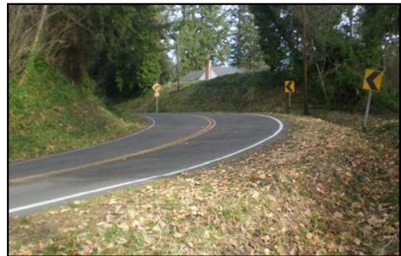
Figure 1.14: East Roadway Curve on SE Mud Mountain Road
