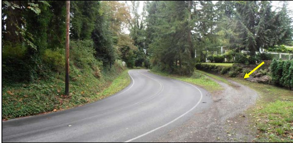
Figure 1.21: Existing Northern Driveway Entrance
