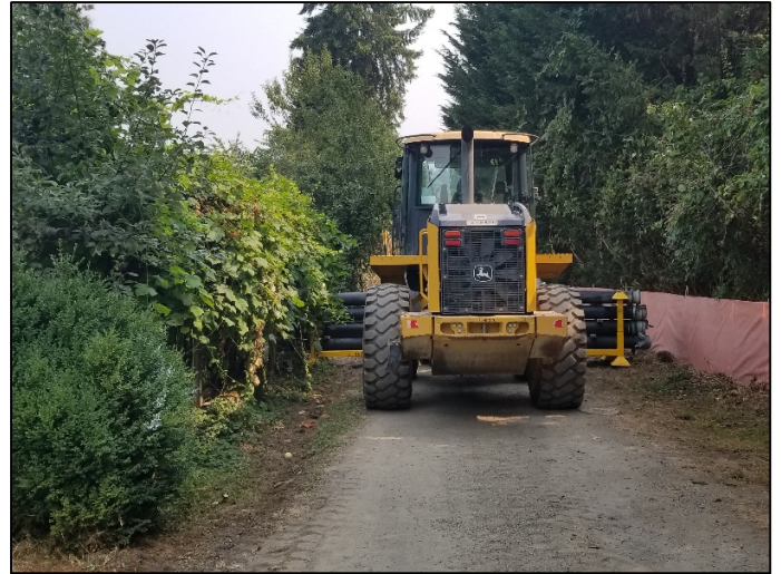
Loader moving pipe thru the constrained corridor to equipment storage location prior to clearing.
