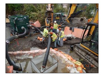
With the City of Sammamish project to replace the culvert under the Parkway nearly complete, the stream bypass system is moved onto the ELST side of the Parkway culvert.
