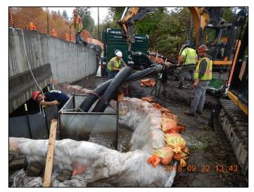
Workers adjust the Zackuse Creek dewatering and stream bypass system between the East Lake Sammamish Parkway and ELST.
