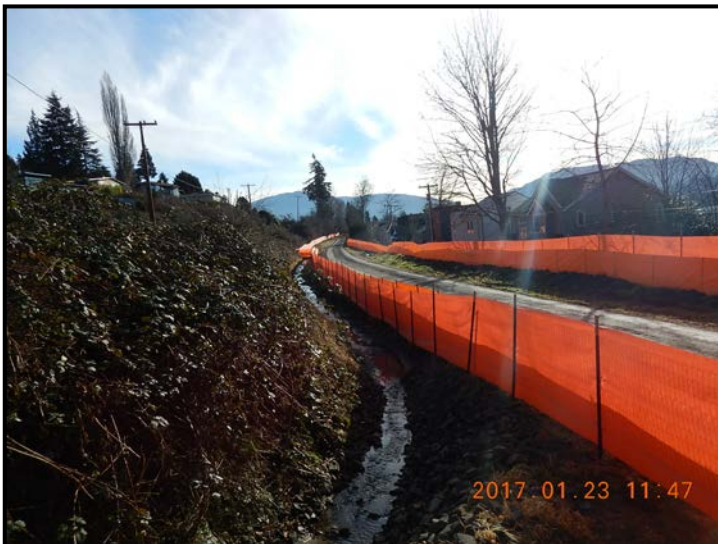
Erosion Control and Safety Fencing
