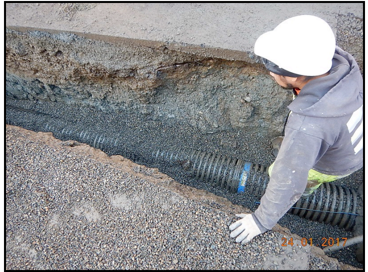
Installation of stormwater pipe
