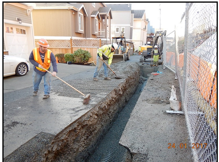
Installation of stormwater pipe
