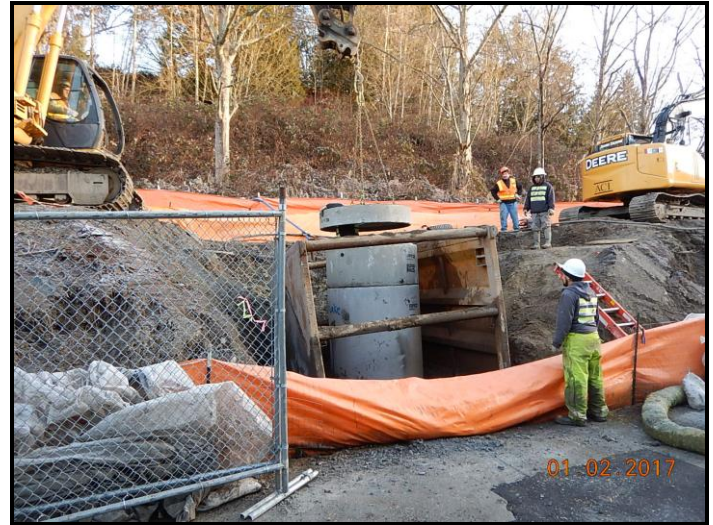
Installing Catch Basin
