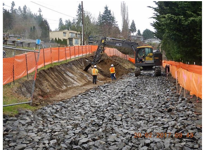
Sta 40+00 - Channel excavation
