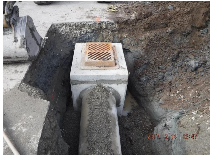
Installing stormwater pipe and catch basin
